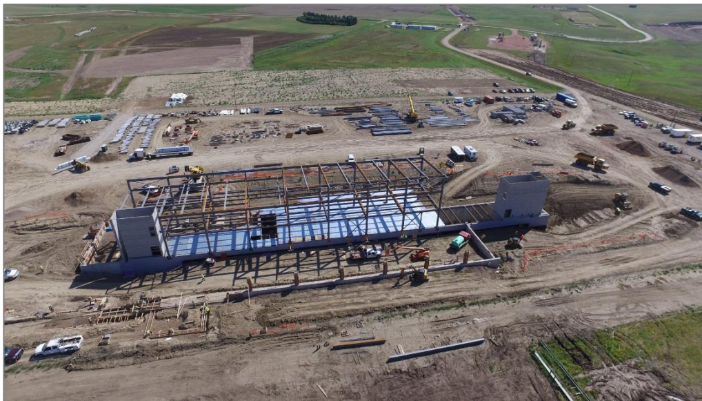
Commercial Terminal Looking East
