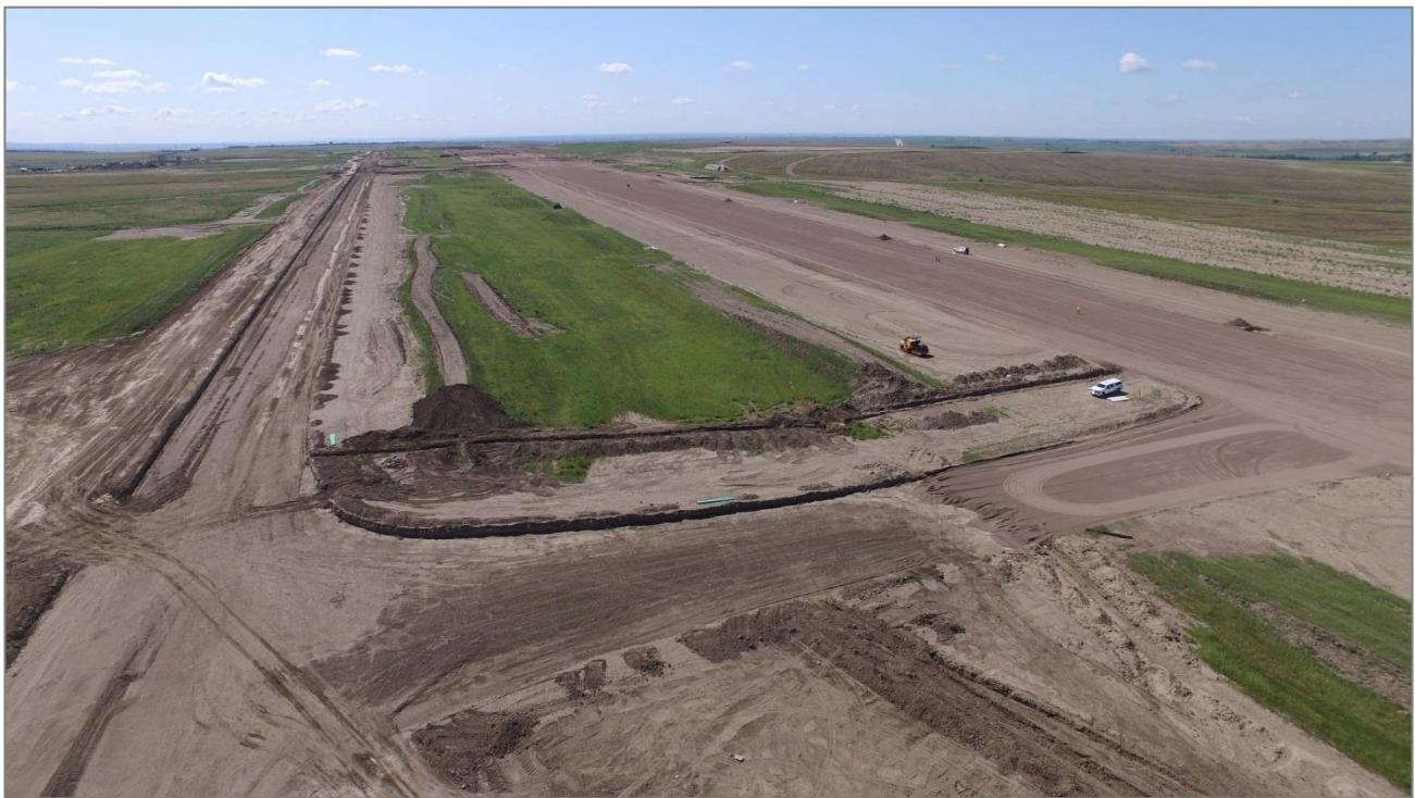
Runway 14 32 and Crosswind 4 22 Intersection
