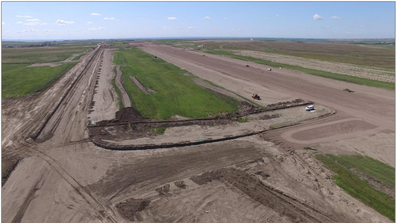
Runway 14 32 and Crosswind 4 22 Intersection
