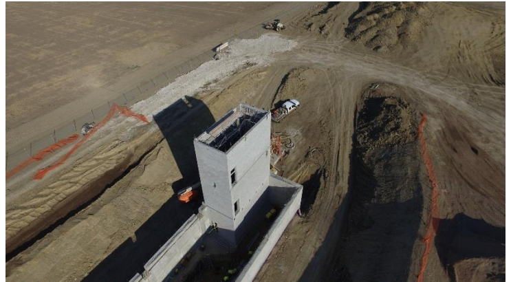
Terminal North Stair Tower
