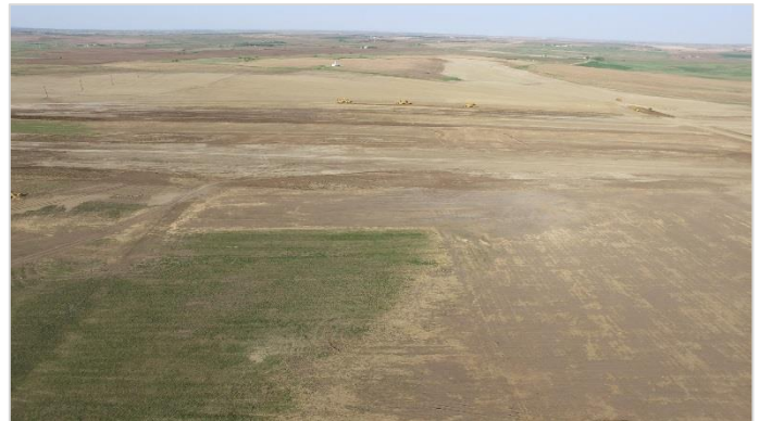
Runway and Taxiway Grading
