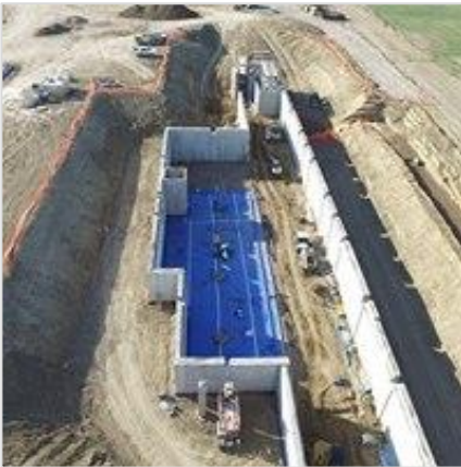
Terminal Basement South Looking North
