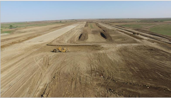
Runway and Taxiway Excavation
