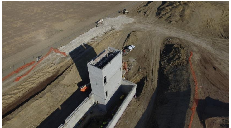
Terminal North Stair Tower
