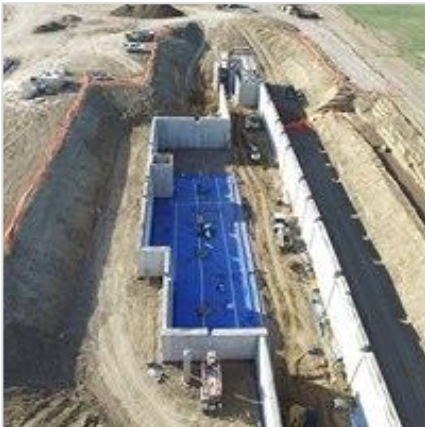
Terminal Basement South Looking North
