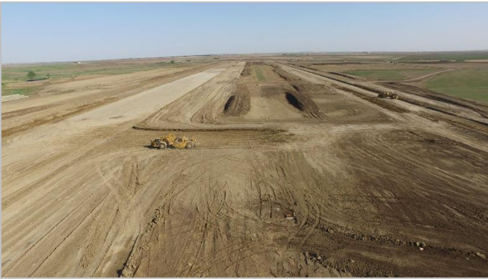
Runway and Taxiway Excavation
