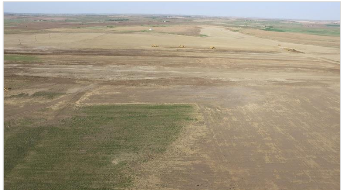
Runway and Taxiway Grading
