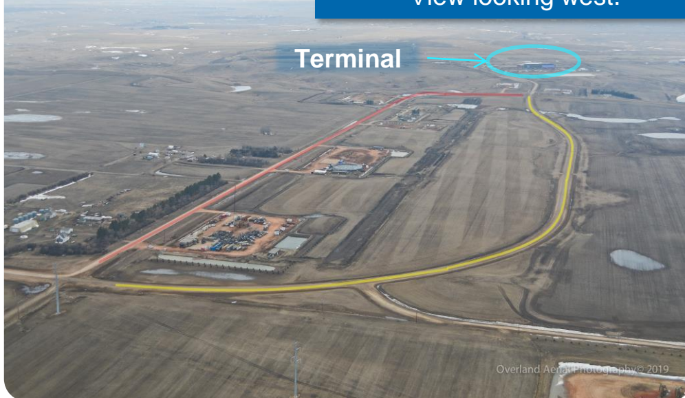
County Road 7 re-routing. View looking west.
