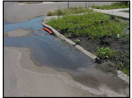
Inlet protection installed correctly
